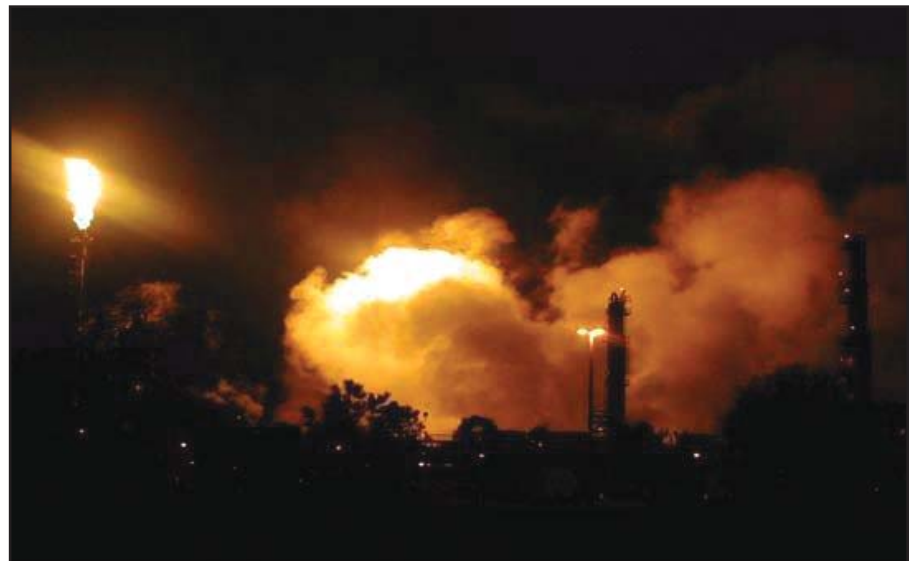
The Conoco Phillips oil refinery is one of several facilities that release massive quantities of pollution and dioxins in Mossville.
